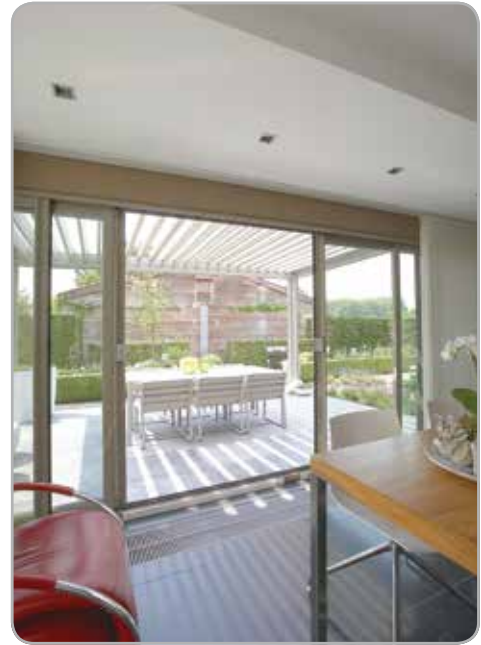
Integrated vertical windresistant sun protection screen based on Fixscreen® technology
